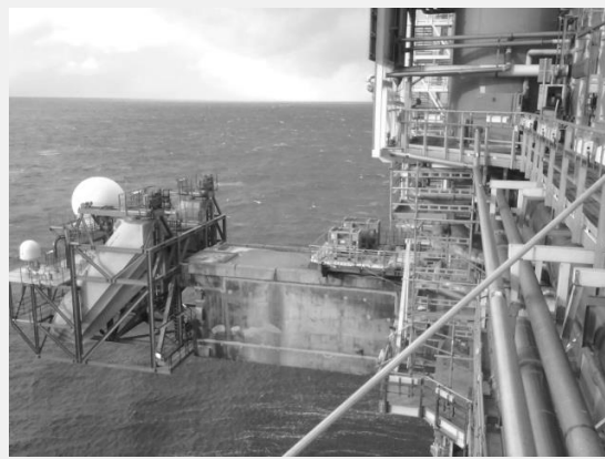
Figure 2. SWCTT location on the Heidrun platform.
